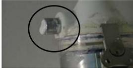
Debris is keeping the filler valve open or valve spring is damaged
