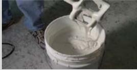
Mix additional joint compound to thicken to desired consistency for internal corner finishing. Remember, mixing joint compound for internal corners generally requires approximately 28 to 32 oz of water per five gallons of Joint compound ready mix material. Check with the joint compound manufacturer for recommended amounts of water to add.
